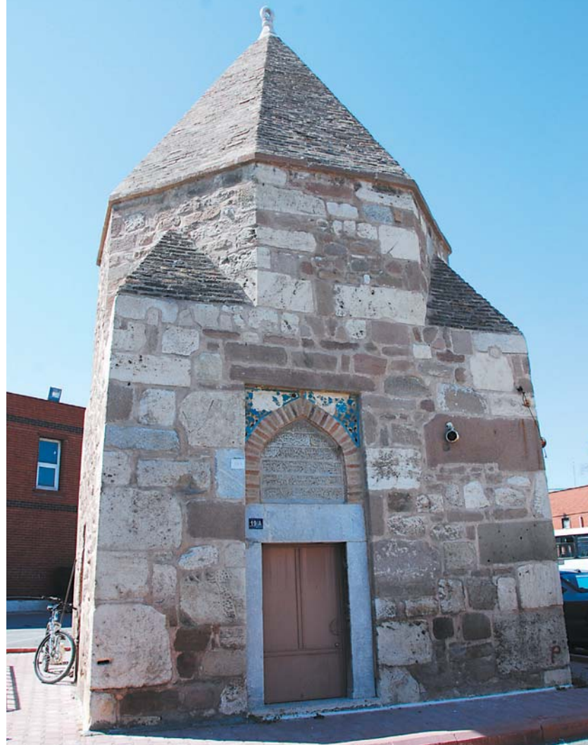
Fakih Dede Tomb, General View / Bey Street Fountain-1, General View
