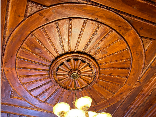
Fotoğraf 35-36: Kız Orta Okulu İç Mekan ve Tavan Süslemesi/ Photo 35-36: Interior and Ceiling Ornamentation of the Girls' Secondary School
